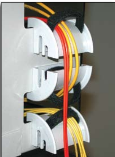
Patch Panel Egress
