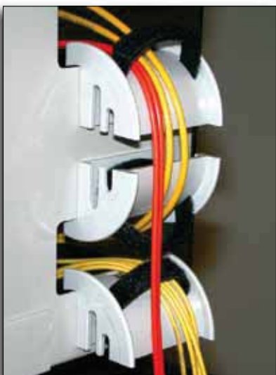
Patch Panel Egress
